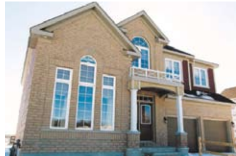
The Platina model uses brick, stone and pre-engineered wood siding to clad the exterior. Solar panels are attached to the roof and to the rear wall of the home.
